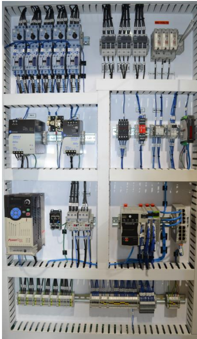
Figure 3 - Typical DensiMAX Control Panel
